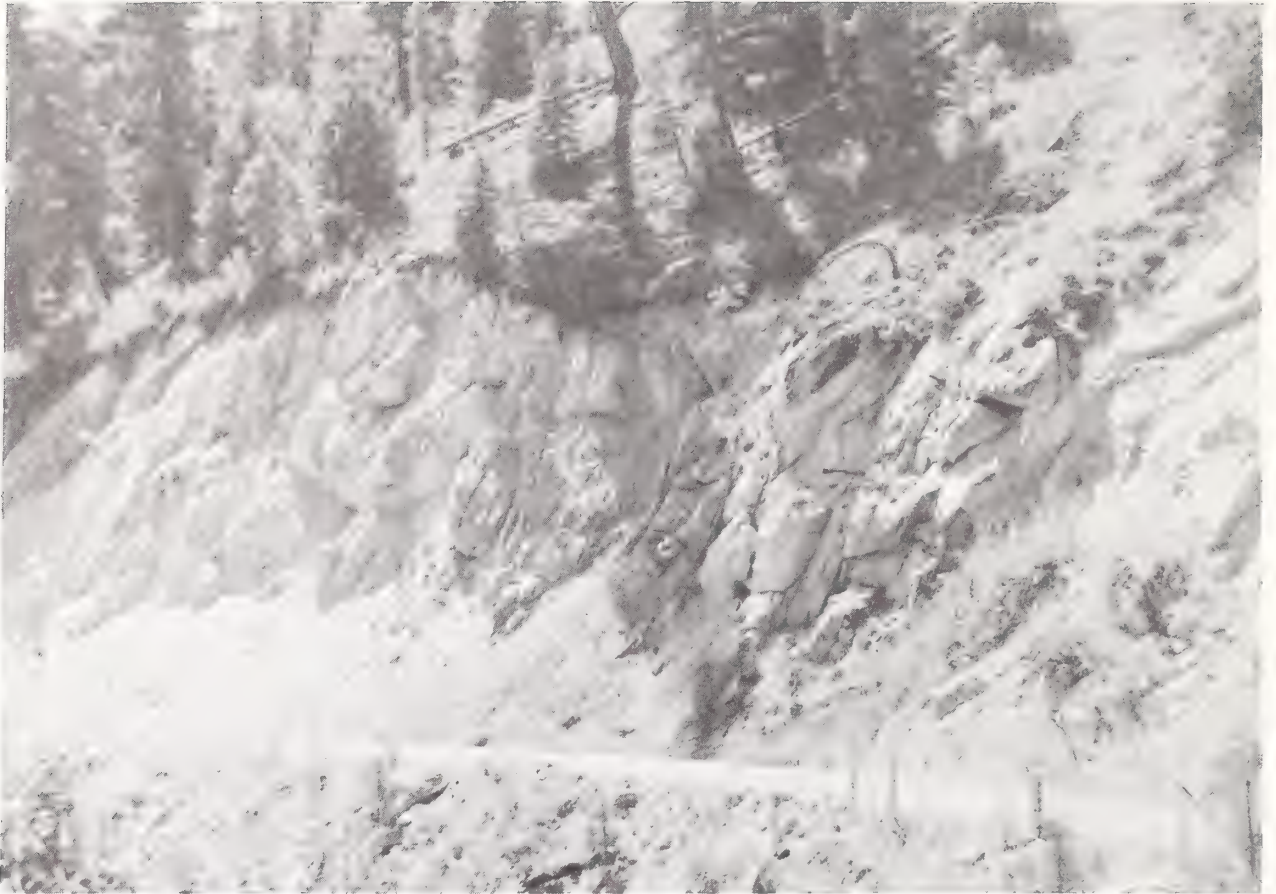
Figure 7.--Granitic rocks in the Idaho Batholith exhibit various degrees of weathering. Road cuts in the more highly weathered types continue to supply sediment for years.
